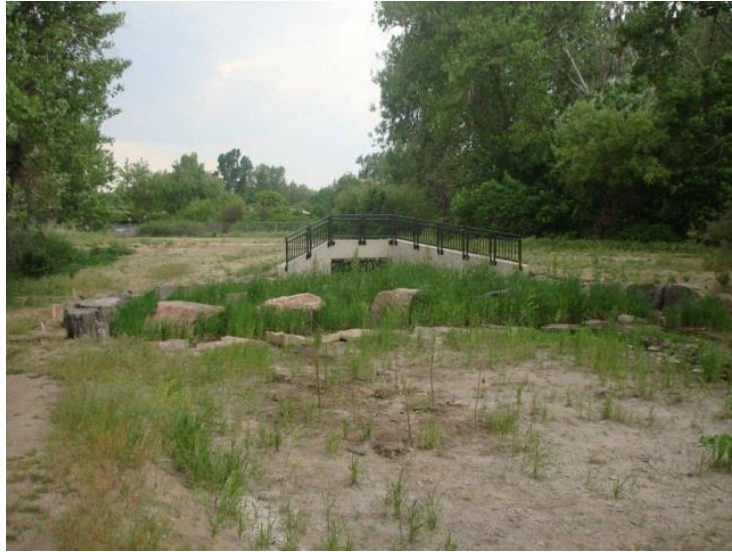
Figure G-2: Application of soil rip-rap at a stormwater outfall.
