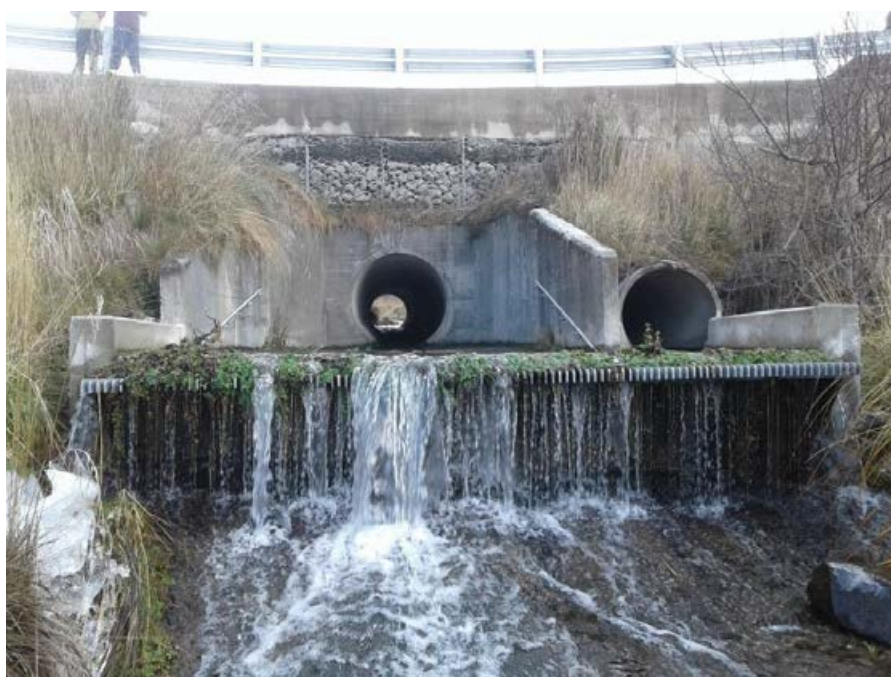
Figure 6-7: An example of an anti-jump screen/ grill that could be added to a barrier to prevent trout access. Photo credit: Sjaan Bowie.
