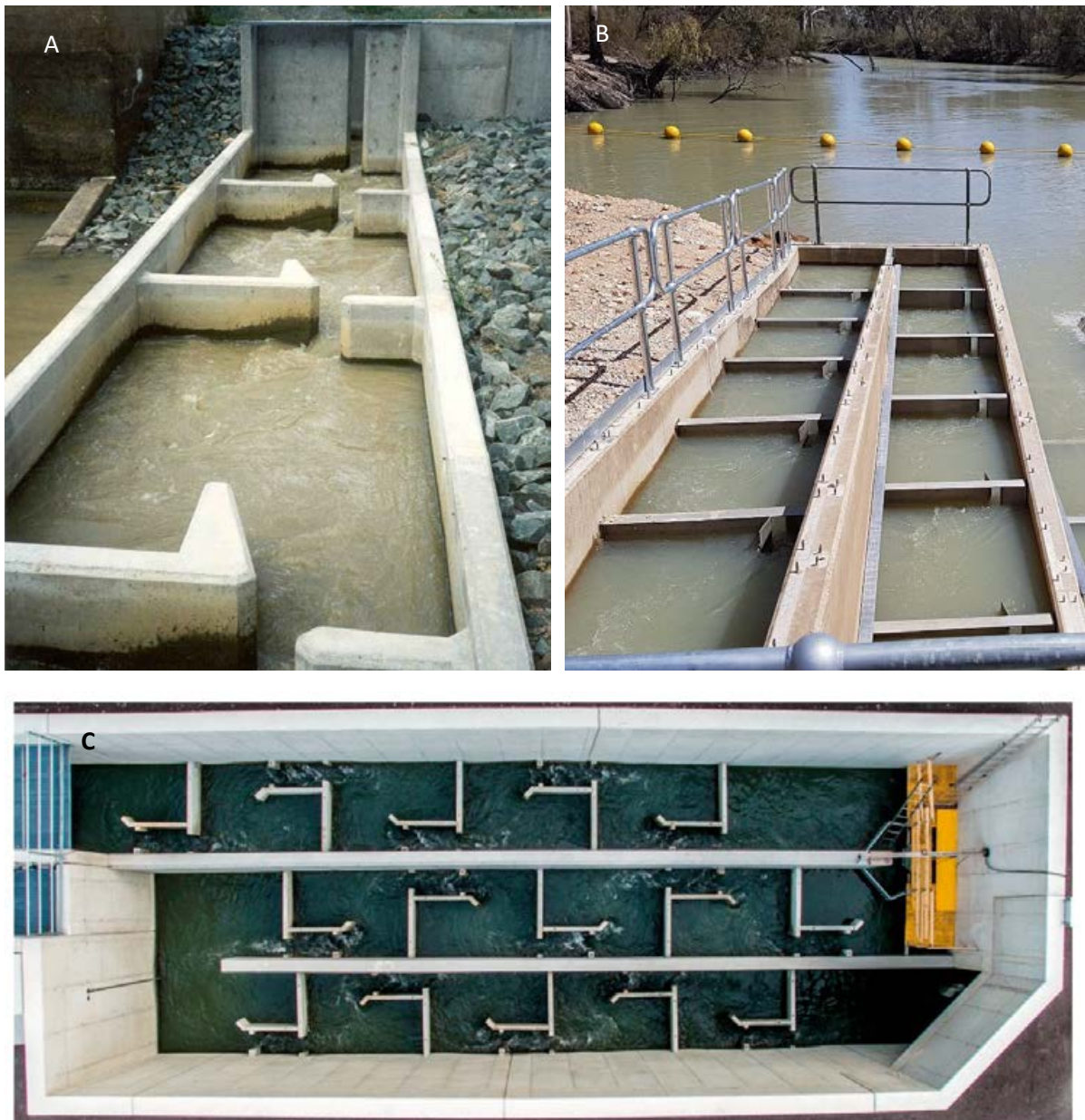
Figure 7-19: Examples of different vertical slot fishway types. A = regular vertical slot fishway (Photo credit Ivor Stuart), B = dual/ multi slot fishway (Photo credit: Tim Marsden), C = E-nature vertical slot fishway (Reproduced from Mader et al. (2020)).
