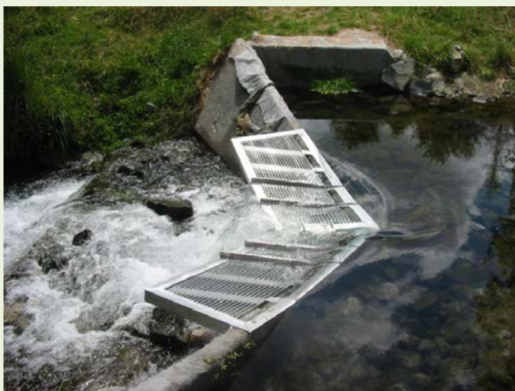
Figure 6-9: Trout barrier at Hamurana Springs. Photo credit: Andy Woolhouse.
