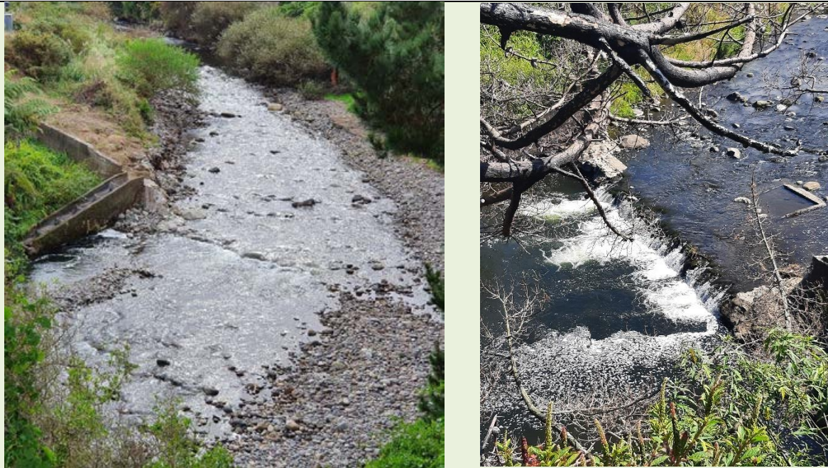
Figure 5-5: The site immediately following weir removal (Left) and two years later showing the 1 m high barrier caused by leaving the weir footings in place (Right). Photo credits: Te Korowai o Ngāruahine (left), Finnley Binsbergen (right).
