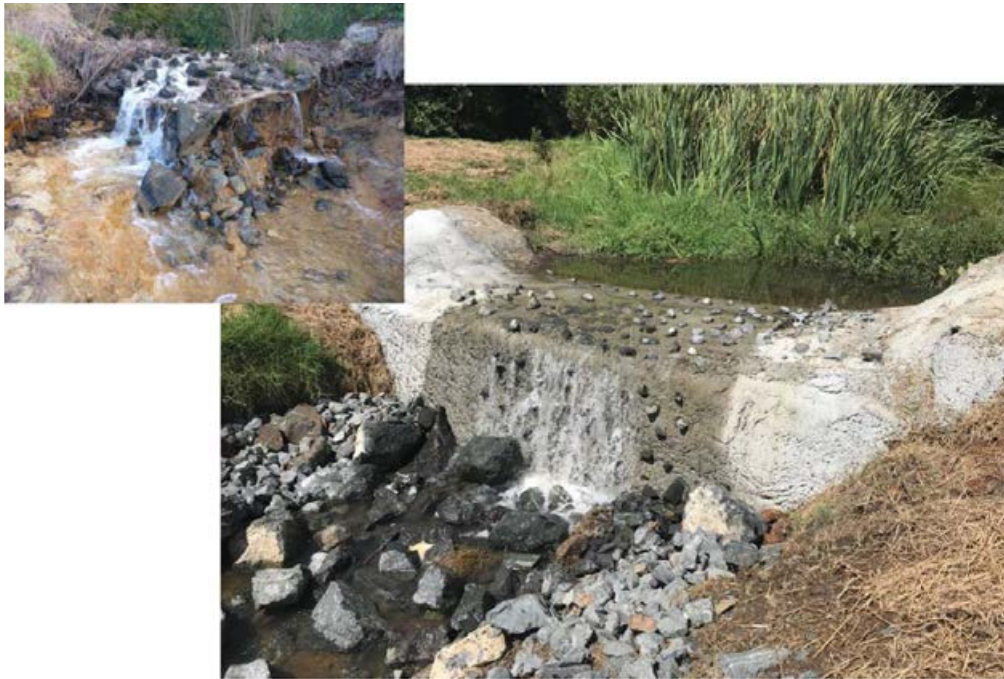
Figure 6-15: Baffled concrete weir in the lower reaches of Puketirini Stream, Waikato. A degraded weir (inset top left) was successfully preventing koi/amur carp, goldfish, perch, rudd and gambusia from accessing upstream habitats while allowing the passage of banded and giant kōkopu, and shortfin and longfin eels. To continue protecting native fish populations, the weir was remediated in 2018. Key features of the barrier include the roughness and wetted margins that desirable fish use to migrate, coupled with shallow water depths at the base of the weir to prevent large-bodied fish jumping Photo credit: Cindy Baker.
