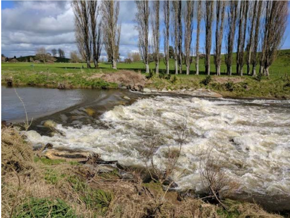
Figure 4-23: A rock ramp style weir on the Waipa River at Otorohanga that also has a fish pass along the true left bank. The fish pass provides passage at low flows when the large rocks forming the downstream face of the weir are exposed and swimming species cannot surmount the weir. Photo credit: Eleanor Gee.
