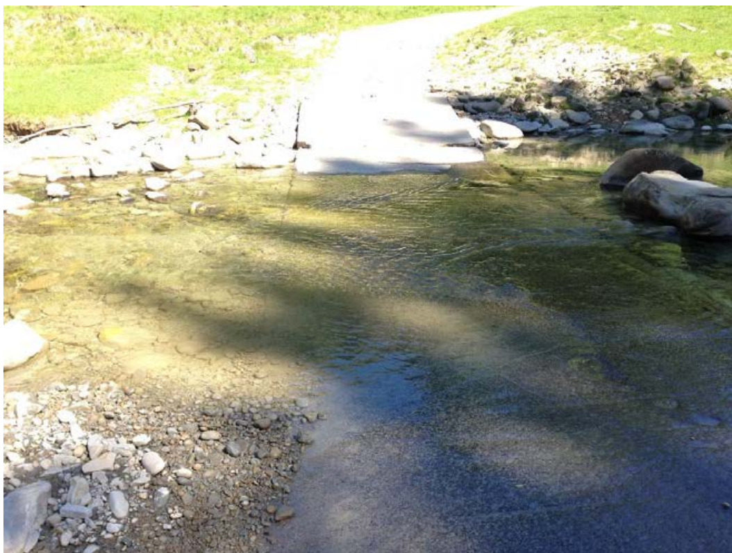
Figure 4-20: Low profile ford crossing.
