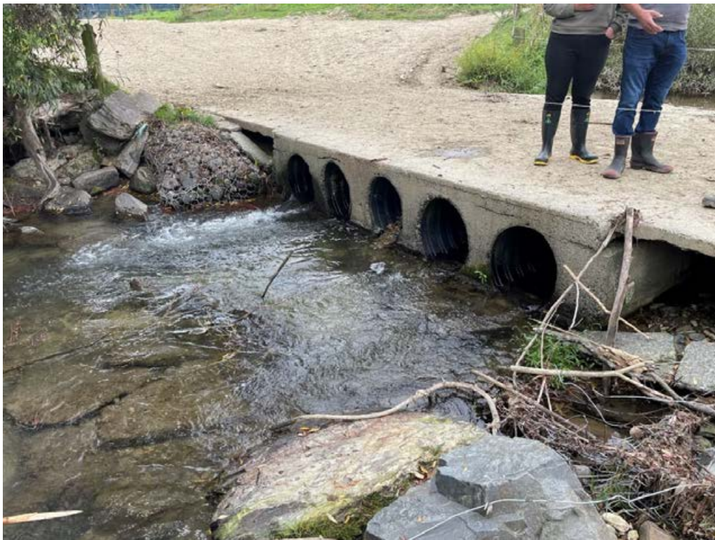
Figure 4-22: Raised roadway ford crossing with culverts. At low flows, water passes through the culverts in the ford, rather than over the roadway. The small culverts used in this ford severely constrict the river channel and will result in accelerated water velocities through the culvert barrel that may be impassable to fish.
