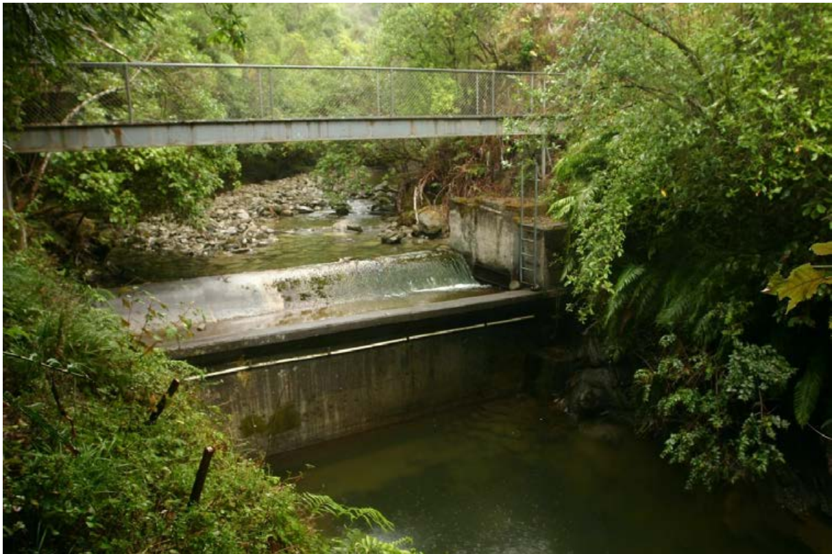
Figure B-7: An intake weir that blocks fish migrations on the Te Arai River near Gisborne. Photo credit: Jamie Foxley.
