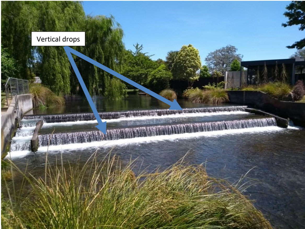
Figure B-13: Example of a weir in central Christchurch. Fish passage will be impeded by the fall height of the steps in the weir and the salmonid fish passes. Photo credit: Megan Brown.
