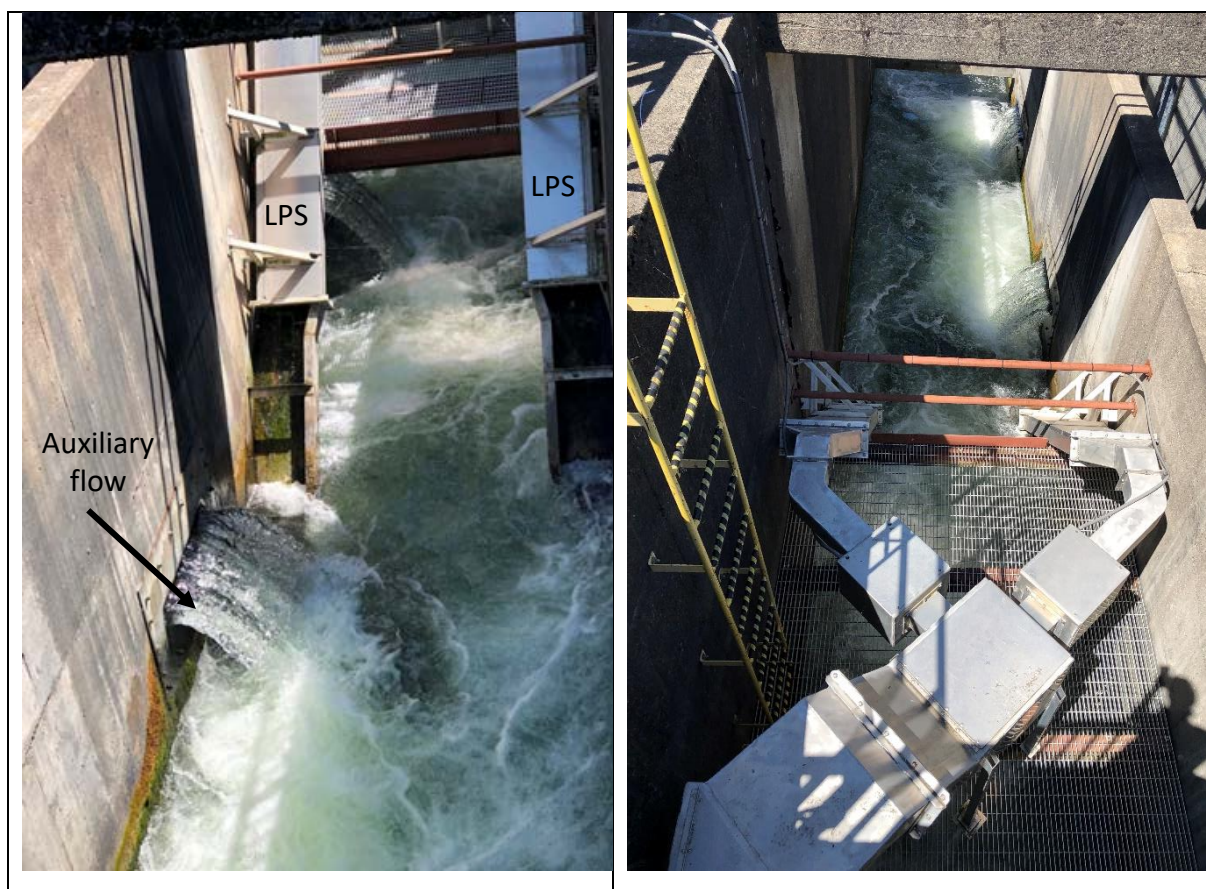
Figure 7-8: Lamprey passage structure (LPS) installed at Bonneville Dam, Columbia River, Oregon. Photo credit: Cindy Baker.
