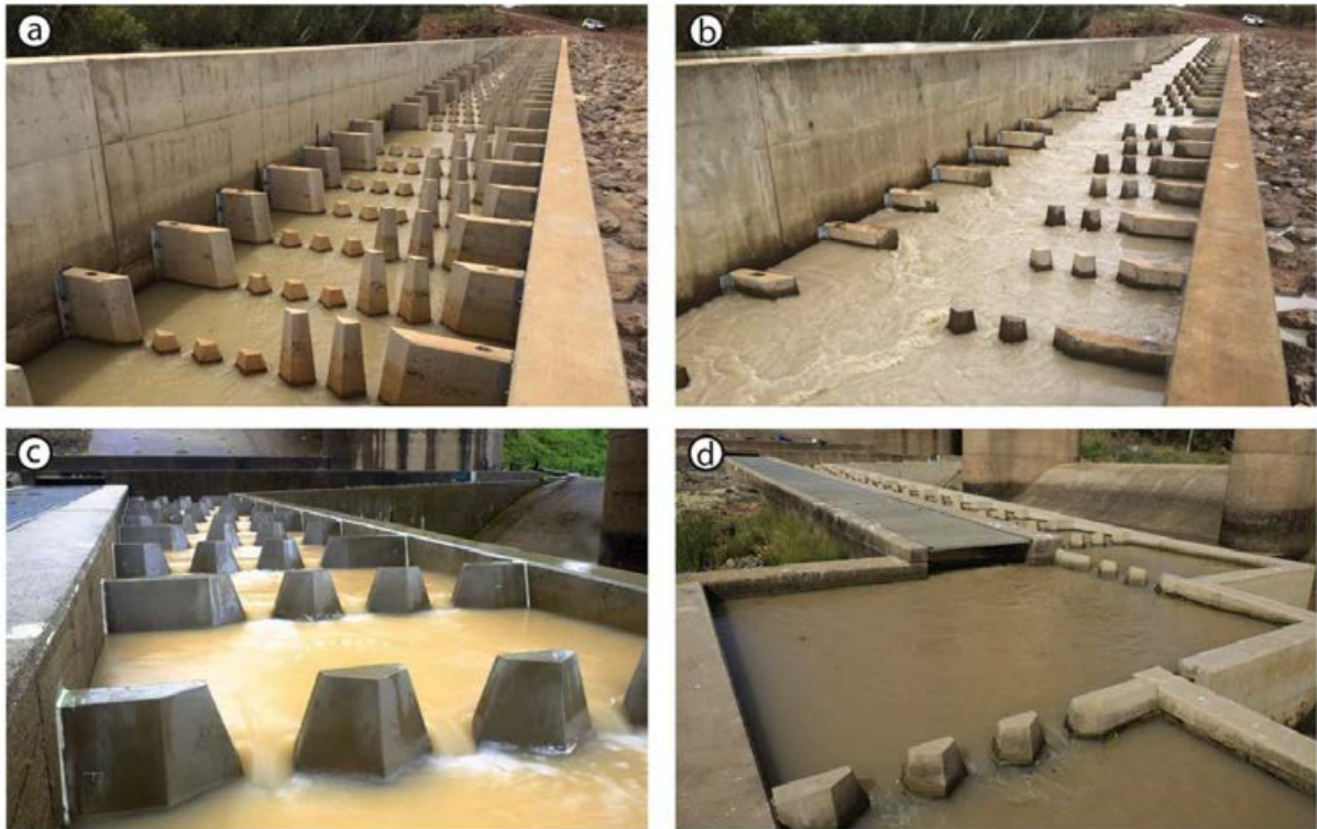
Figure 7-21: Examples of cone fishways. Panel a) and b) shows a high/low cone bypass (at Glenore weir fishway) at high and low flows. Panel c) shows a low cone bypass at the Fitzroy River Australia and d) is a tailwater stabilisation pool which improves hydraulics. Source: Stuart and Marsden (2021).
