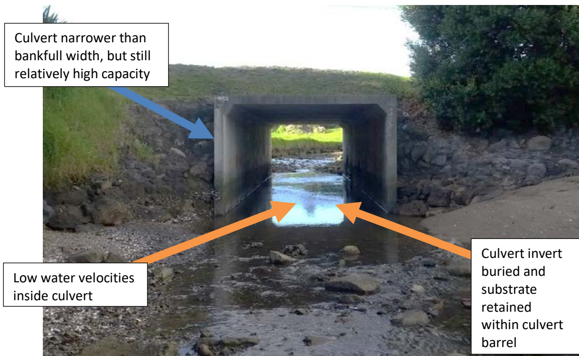
Figure B-22: Example of a culvert in a tidally influenced area. The culvert invert is embedded meaning that natural substrate is retained through the culvert. Culvert width relative to the stream bankfull width is lower than recommended, but because the culvert is in a tidal area, low water velocities will exist through the culvert during slack tide conditions. Photo credit: Bryn Quilter.
