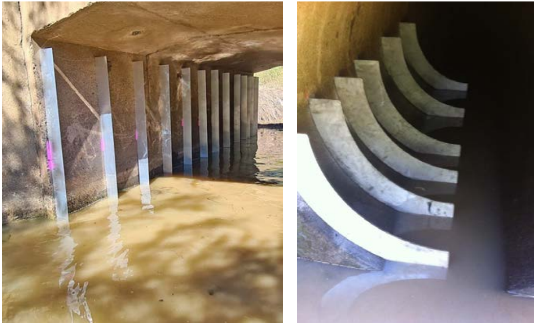
Figure J-3: Examples of vertical baffles. Photo credit: Tim Marsden, Australasian Fish Passage Services.
