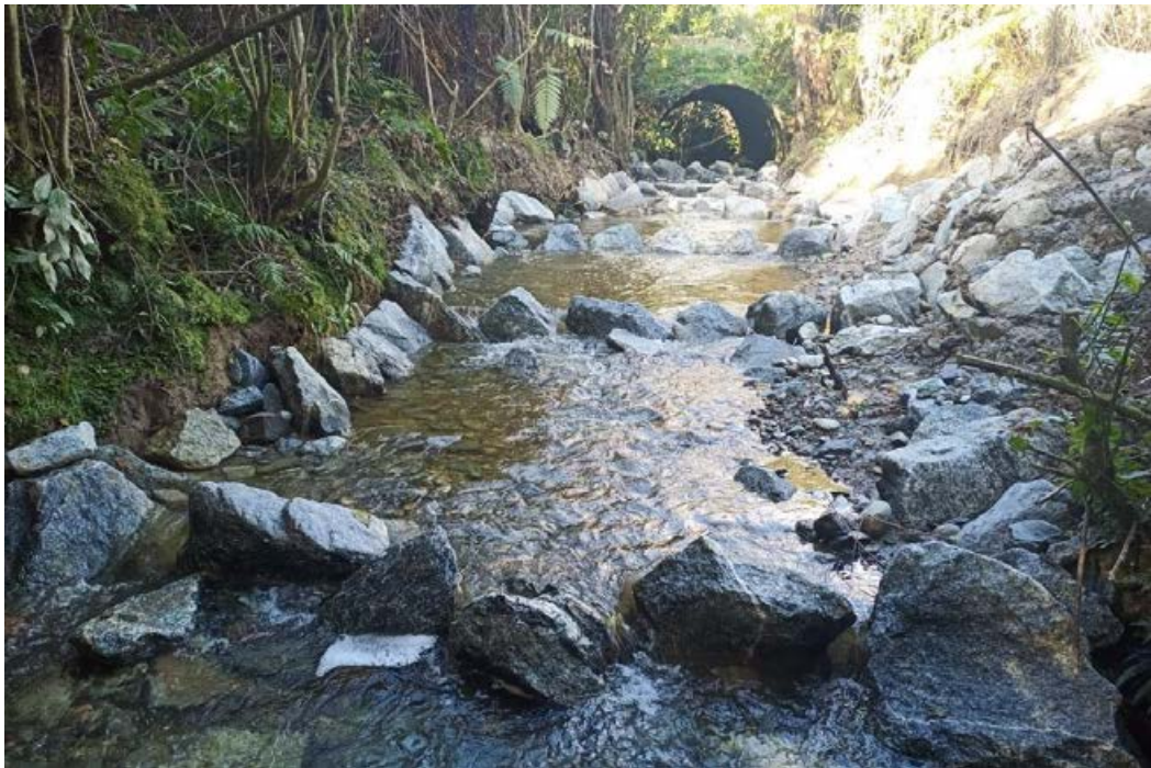
Figure 5-9: Example of a full-width rock ramp fishway in Mill Creek, West Coast. Photo credit: Koen Beets.
