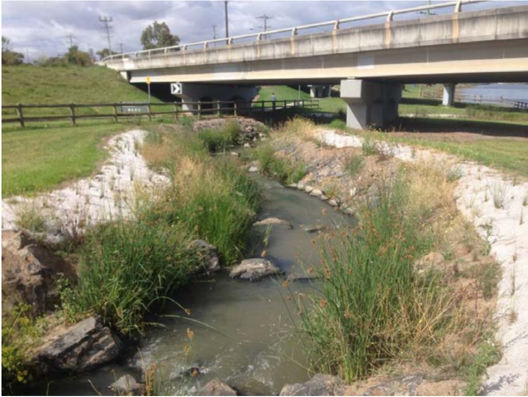
Figure 5-8: Example of a small low gradient nature-like rock ramp fishway on the Patterson River near Melbourne, Australia. Photo credit: Paul Franklin.
