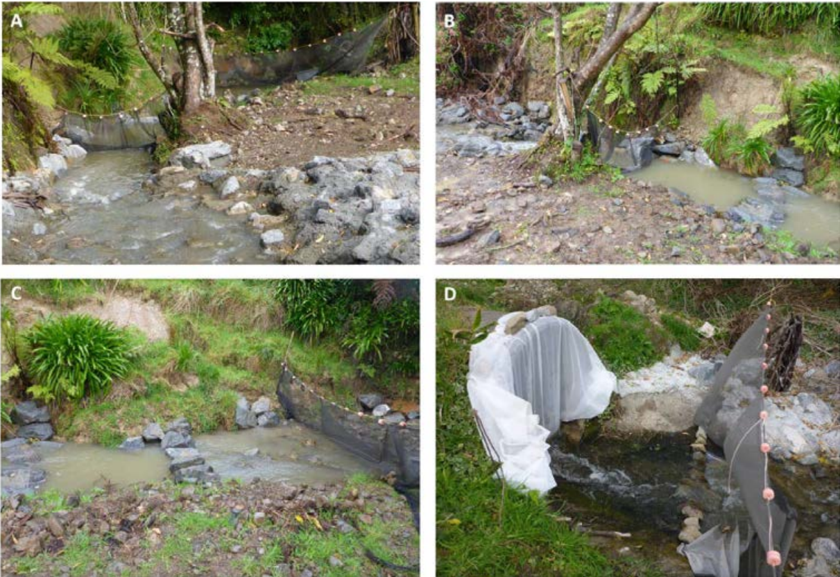
Figure 8-12: Downstream barricades installed in Kara Stream during the inanga passage trial. A - C Barrier nets deployed during the rock ramp trial. D, Barrier nets deployed for testing inanga passage through the culvert independently of the rock ramp.
