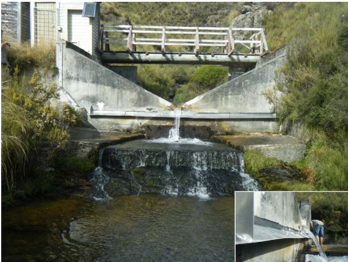
Figure 6-13: Full exclusion barrier installed in an un-named tributary of Upper Waipori River. The objective was to prevent trout and kōaro access to a key dusky galaxias stronghold in Otago. Inset shows a close-up view of the successful kōaro lip barrier. Key features of the barrier include the 175 mm depth aluminium sheet with 100 mm angle, sealed to the weir face with no gaps at a 120 degree downwards angle. Photo credit: Josh Tabak.
