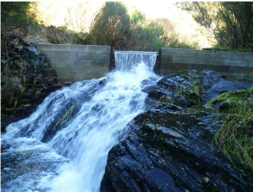
Figure 6-3: Akatore Creek barrier in Otago. A high head exclusion barrier installed onto a natural waterfall to protect Taieri flathead galaxias, after brown trout gained access upstream when conditions changed at the natural waterfall. Key features of the barrier are the height to prevent trout access, the overflow to minimise backwater creation and loss of non-migratory galaxiid habitat, and the wood boards to manage height and enable flushing if required. Photo credit: Sjaan Bowie.
