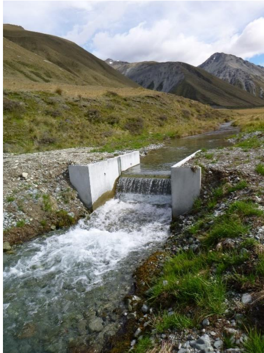
Figure 6-4: High head exclusion barrier installed in Fork Stream, Canterbury. The barrier was built to prevent trout accessing a key non-migratory galaxias stronghold in Fork Stream, Upper Waitaki River, Canterbury. Key features of the barrier were the height and downstream shallow zone (concrete splash pad) to prevent trout access, and the adjustable boards that can be slotted in and out to flush the habitat, minimise backwater and increase height if needed. Photo credit: Sjaan Bowie.
