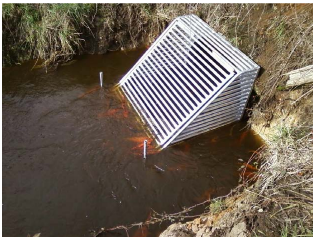
Figure 6-11: One-way gate fitted to Lake Ohinewai outlet drain, Waikato. The objective was to establish a selective exclusion barrier to prevent large koi/amur carp from migrating upstream into the lake, while allowing juvenile native species to move upstream, and all fish to move downstream to exit the lake. Photo credit: Adam Daniel.
