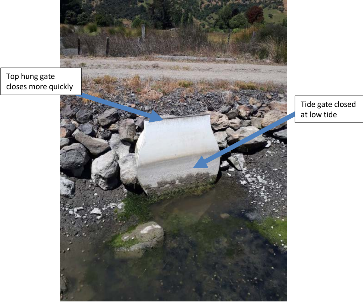
Figure B-14: Example of a culvert with a flap gate. Fish passage will be impeded by the flap gate being closed, even at low tide. Photo credit: Sam Ammon.
