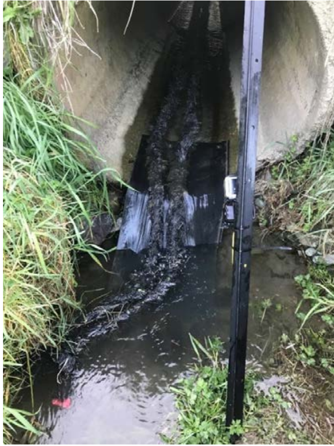
Figure I-1: Example of a rubber ramp deployed at a perched culvert in combination with mussel spat ropes.
