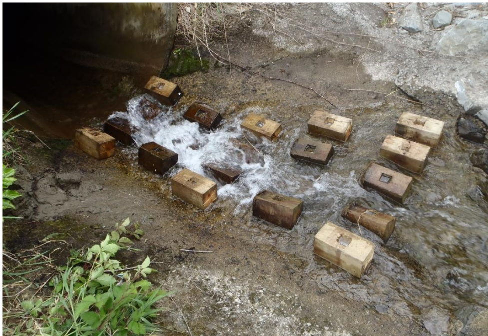
Figure B-4: Rectangular spoiler baffles anchored to the Upper Kingston Road culvert apron.
