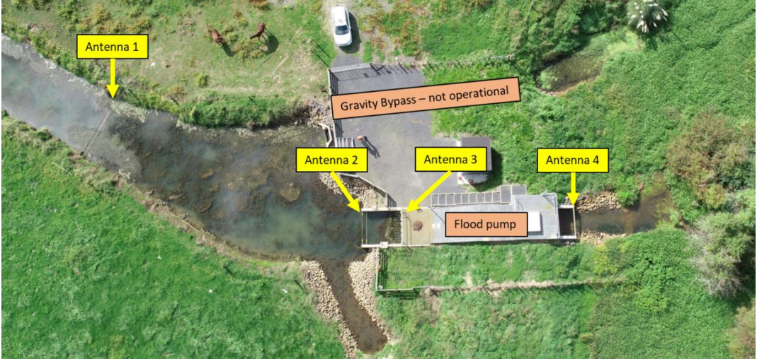
Figure 6-16: Passive Integrated Transponder (PIT) antenna setup at a flood pump station without an operational gravity bypass. Figure modified from Mahlum et al. (2023). Photo courtesy of Waikato Regional Council. Flow moves from the left to the right of the picture.
