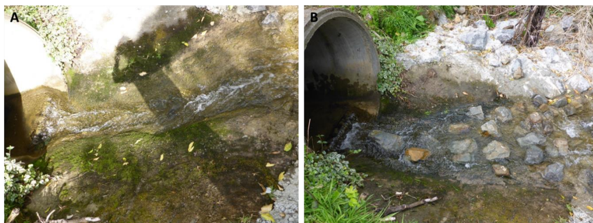
Figure B-3: Culvert apron at Upper Kingston Road. A) unmodified. B) modified using boulders as baffling elements.
