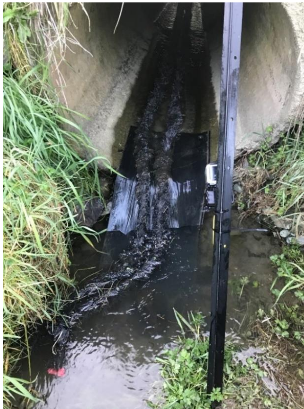
Figure A-1: Rubber ramp and spat rope installed at the outlet of a perched culvert on an unnamed tributary of Oldham Creek, Atawhai, Nelson.
