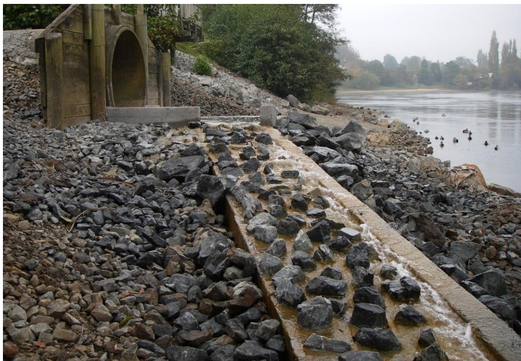
Figure D-1: The receiving pool and fish ramp operating under summer low flow conditions.
