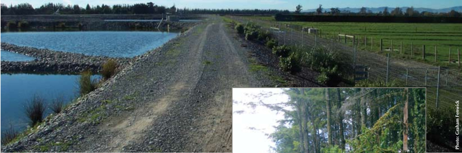
Once treated oxidation pond effluent has been discharged, natural processes render it harmless. Here, treated effluent from oxidation ponds (left) at Leeston, Canterbury, is irrigated onto border-dyked paddocks on the right of the access road. What happens to it once it disappears below the surface is the focus of our research.
