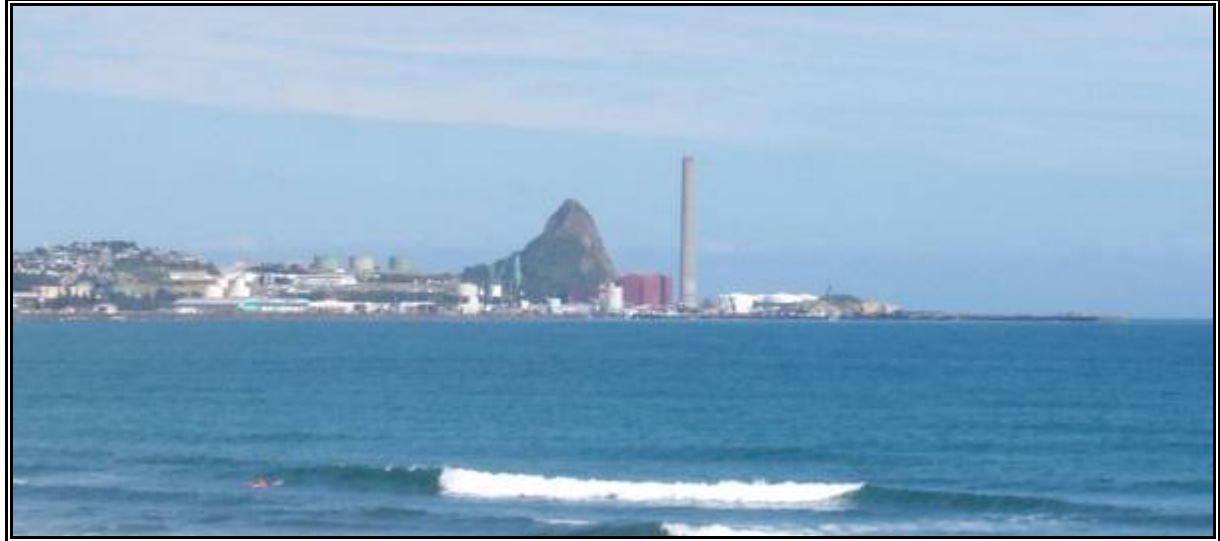
Figure 2-1. The New Plymouth Power Station (view from the northeast).
