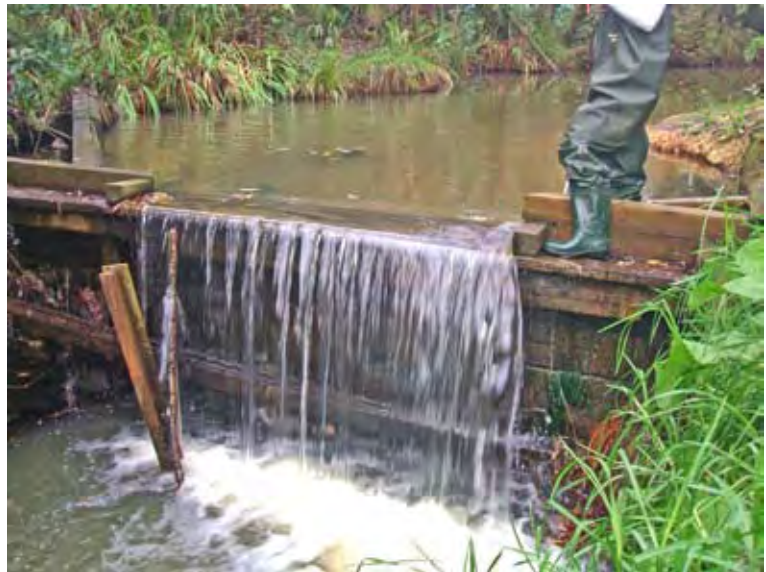
Example of potential barriers to fish passage: dam.
