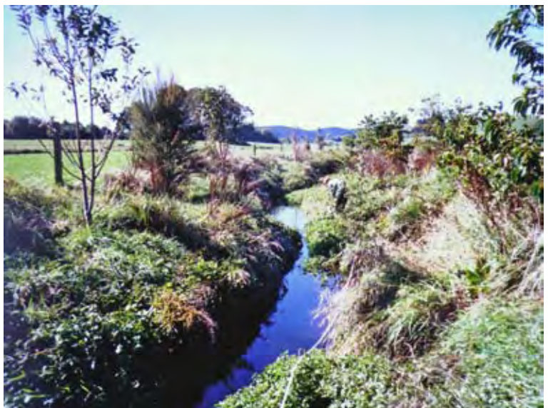
Figure 5.2: Bank damage of a pasture stream in pumice geology (top) and a downstream reach 3 years after fencing and planting (below). Photo: Steph Parkyn
