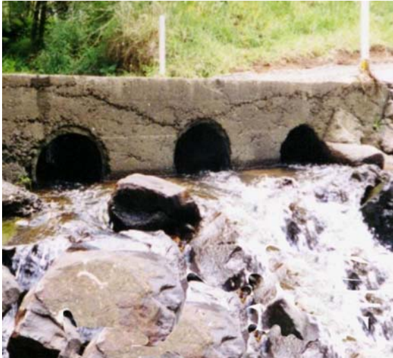
Figure 7: Examples of culverts that prevent upstream passage by inanga.
