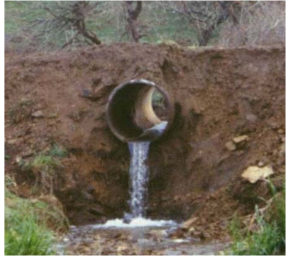
Figure 7: Examples of culverts that prevent upstream passage by inanga.
