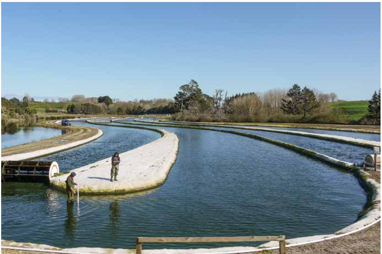
The Cambridge Wastewater Treatment Plant uses NIWA-developed technology to cost-effectively treat, and recover energy and nutrients from, wastewater. (Jason Park)
