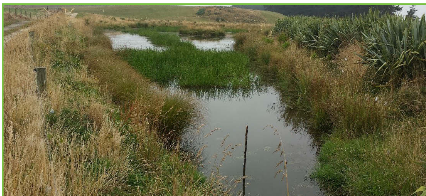
Wetland viewed from the inlet showing emergent beds of kuta and island in the background. Greater plant coverage particularly on the margins would improve the performance of this wetland.
