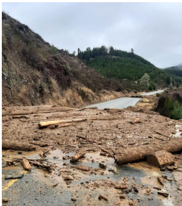
Photo 2: Slips and debris on the road in the Tasman region after heavy rain on 25 July. Credit: Tasman District Council @tasmandc
