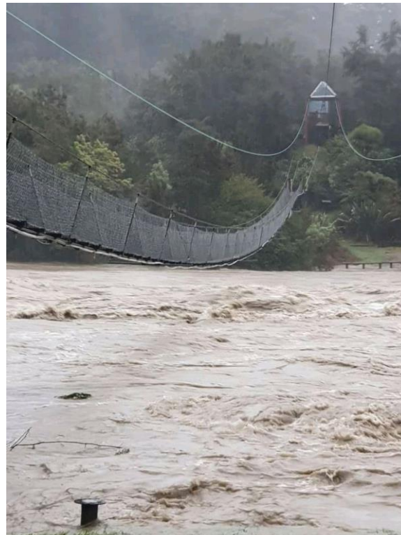
Photo 1: Buller River swing bridge on 17 July.
