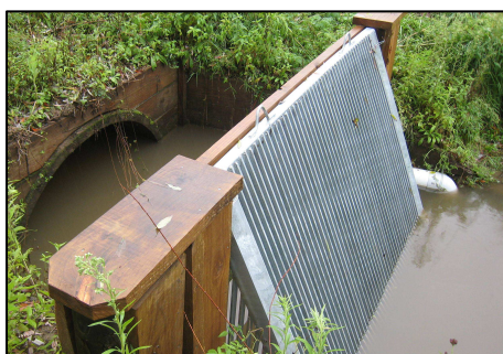
Figure 16: Vertical bar screen to prevent fish emigration from a lake.
