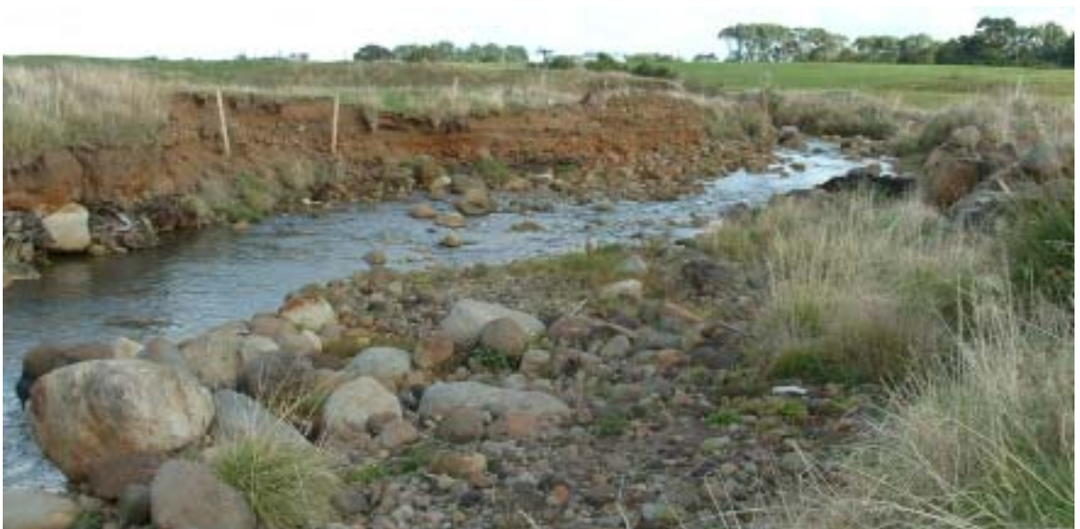
Photo 15 The new channel, 17 months after the stream was diverted (13 May 2009)
