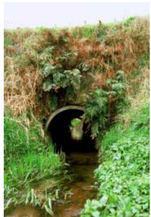
Photo 2 A well designed culvert that will provide for fish passage
