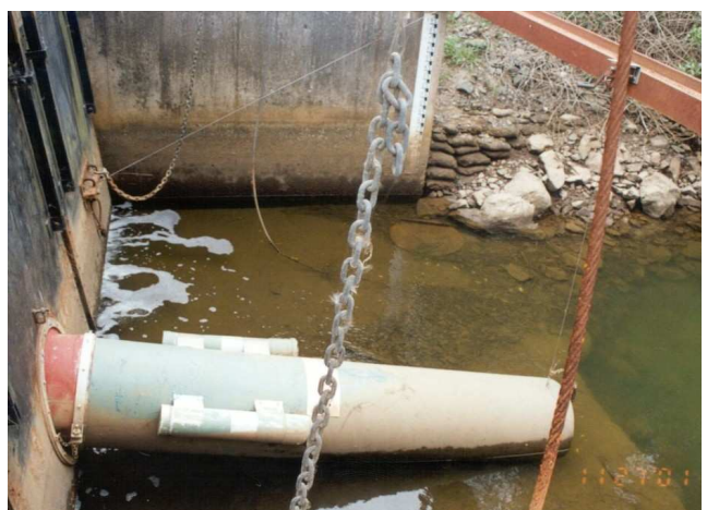
Plate 10 : Liquid levelling regulator
