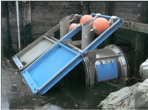
Plate 7: Automatic tide regulated floodgates
