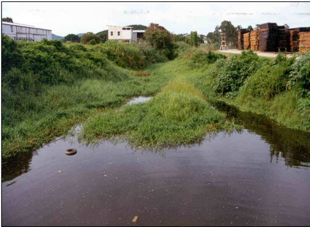
Plate 5: Before active floodgate management, Condong Creek (4/98).
