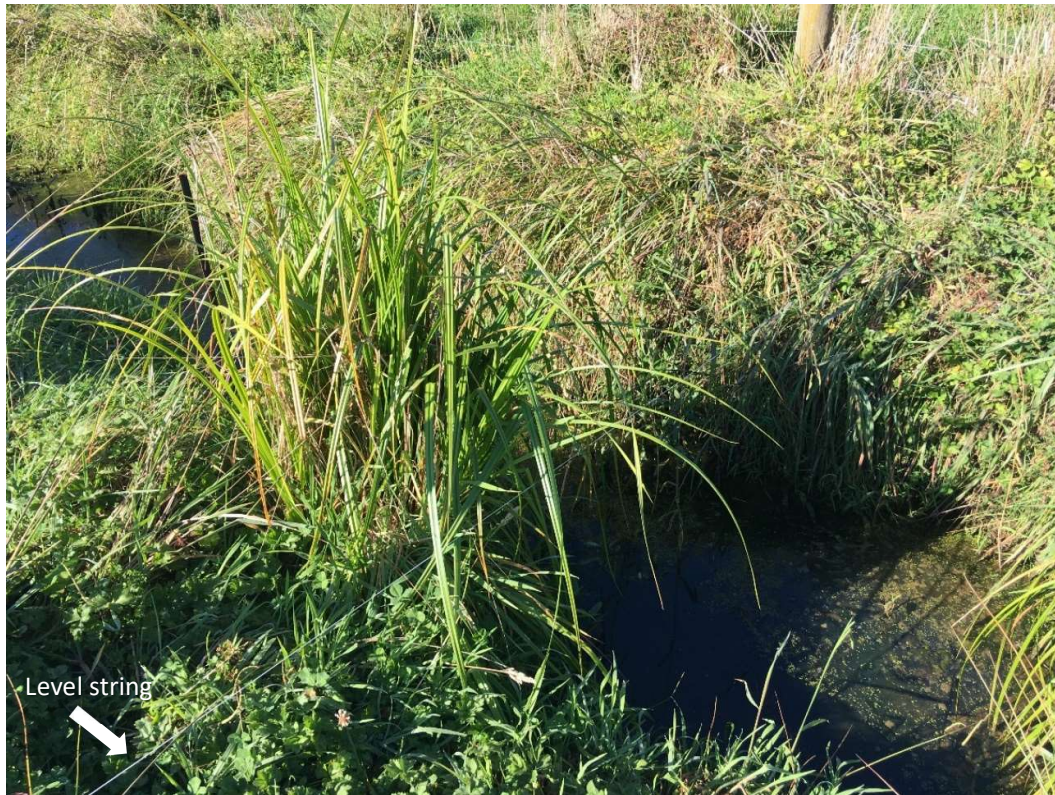
Figure 2-10: Drain at Berry Farm. Level string across the drain is visible beginning bottom left of photo.
