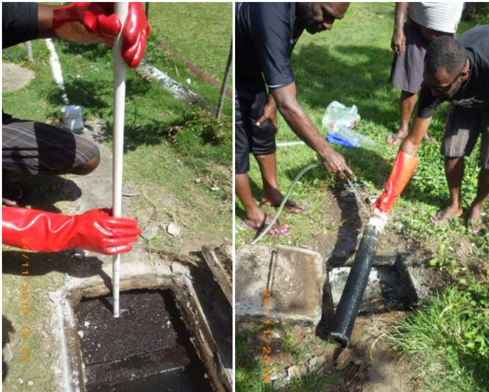
Figure 3-3: Auditing septic tank sludge accumulation. Assessing scum and sludge depths (left) and cleaning septic tank outlet filters (right).
