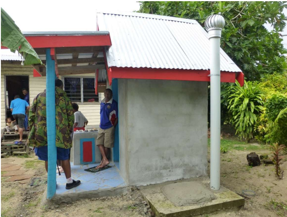
Figure 2-3: ecoVIP2 pit latrine showing vent pipe. Note the pipe has not yet been painted black, necessary to aid convective ventilation.
