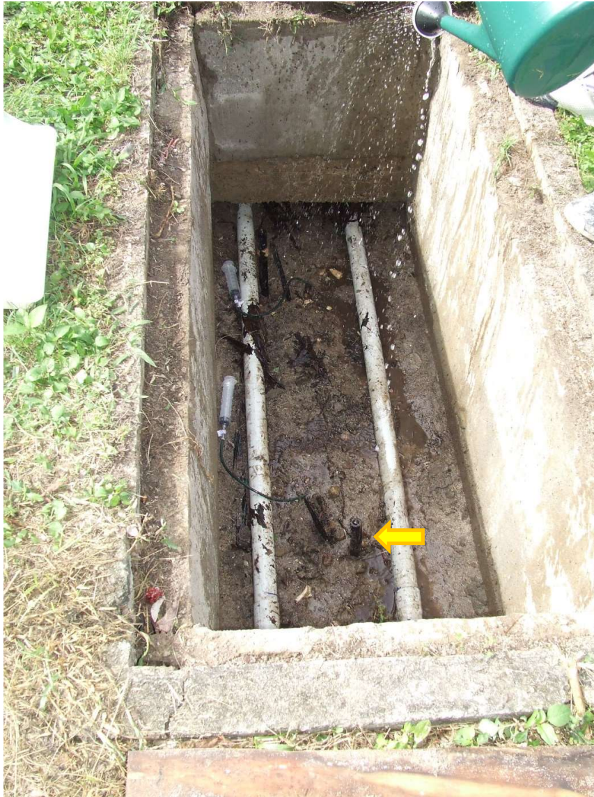
Figure 4-5: Addition of wastewater during system sampling using a watering can. Syringes can be seen attached to the FullStop™ sampling devices (arrowed) to enable samples to be drawn from the base of the bed.
