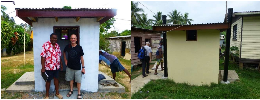
Figure 2-5: ecoVIP2 pit latrine tested in Bavu village. During final stages of construction (left) before ventilation pipes fitted, and from back once completed (right) showing ventilation pipes.
