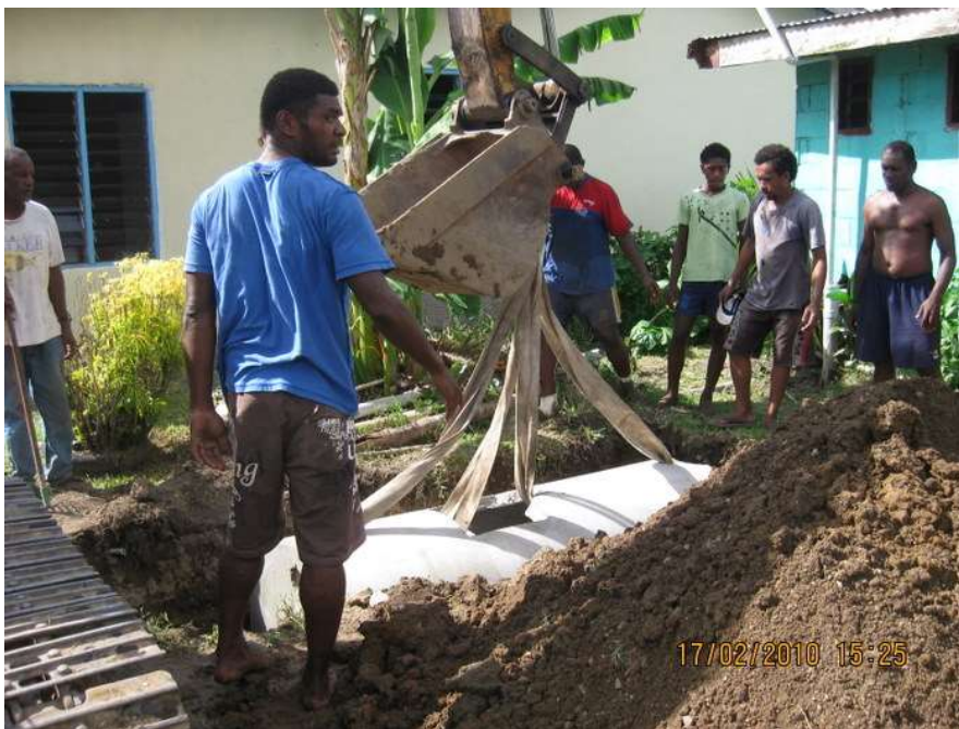
Figure 3-1: New prefabricated septic tanks being installed in Votua village in early 2010.
