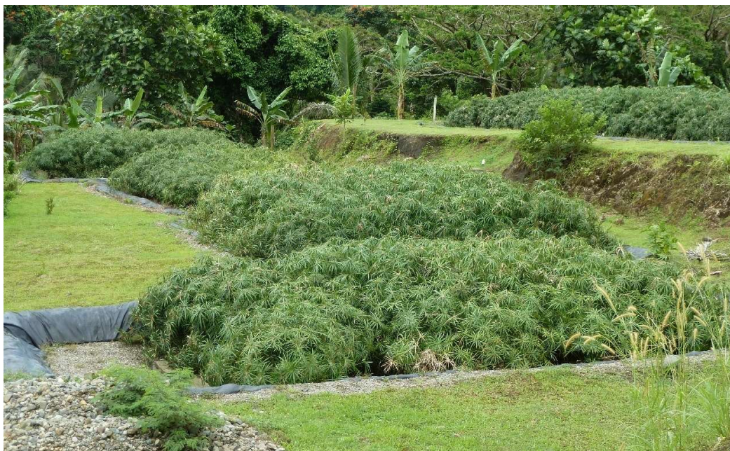
Figure 5-7: The four horizontal-flow wetlands (left) and two vertical-flow wetlands (top right) in April 2011.
