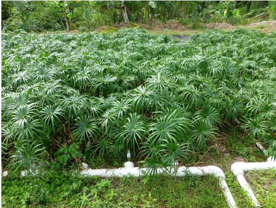
Figure 5-6: Vertical flow wetland vegetated with umbrella sedge. Note dosing pipes which disperse the flow across the surface of the wetland.
