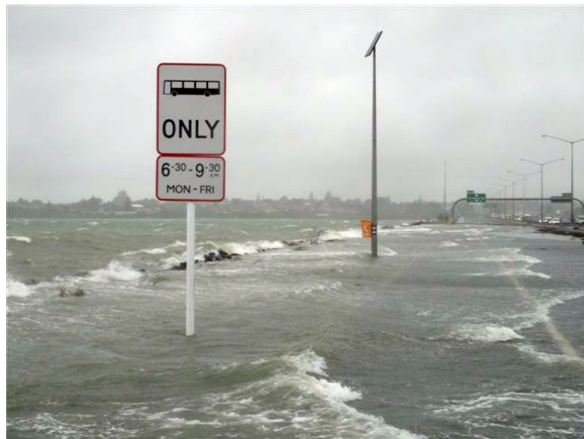
Figure 11. Southbound lanes on Auckland's northern motorway are submerged during a storm that coincided with high tide in January 2011. Source: NZTA
