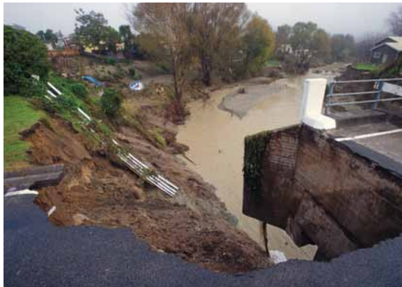
A stream at Waimārama, bloated by three times the region's average April rainfall, seriously damaged this bridge in the small Hawke's Bay settlement. (Dave Hansford)
