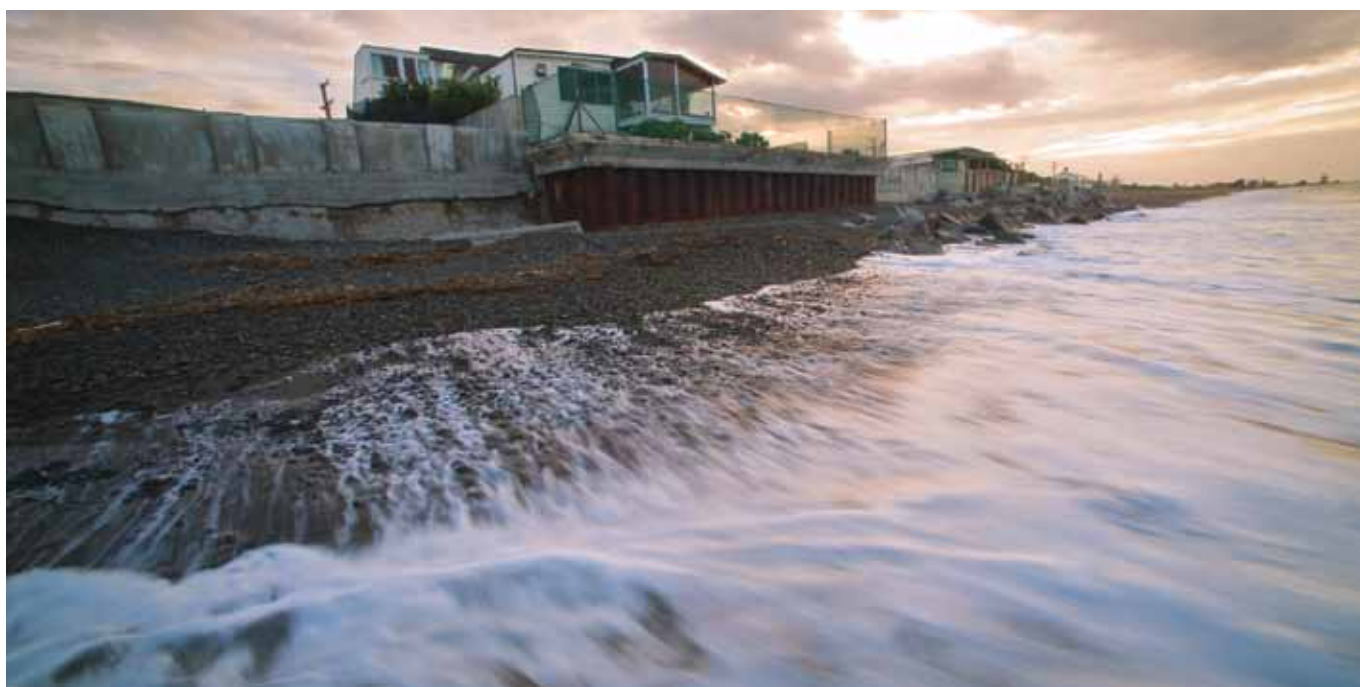
Seafront property owners at Haumoana, on the Hawke's Bay cape coast, routinely flee their homes in the face of waves that break a little closer every year. (Dave Hansford)
