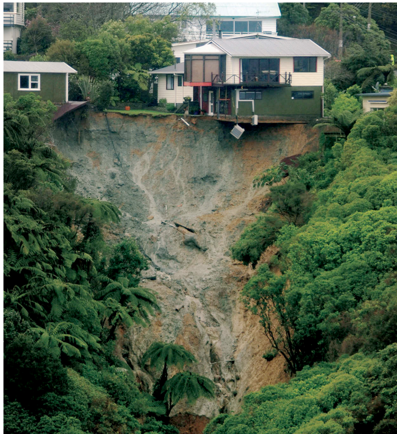
Heavy rain undermined this house at Kelson, Wellington, in a 2006 storm. (Alan Blacklock)
