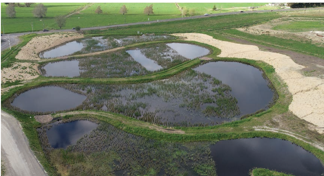
Maniatutu is a series of connected ponds. Deep pools combine with densely planted shallow sections to trap sediment and filter contaminants. (Les Anstis)
