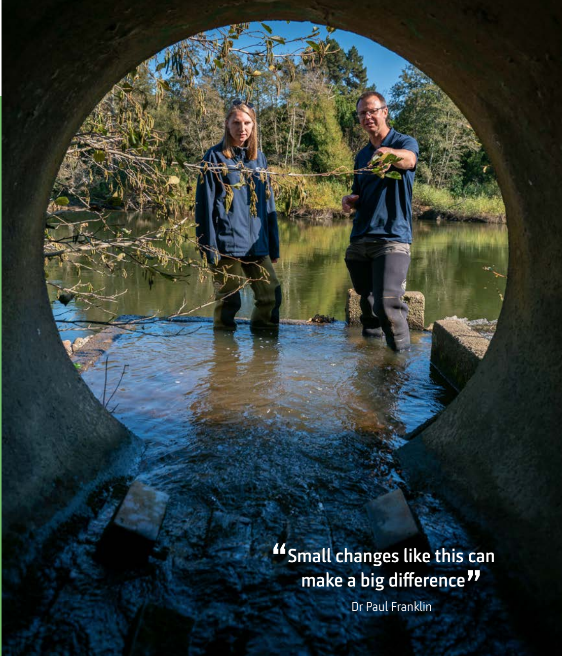
PhD student Rachel Crawford and freshwater ecologist Dr Paul Franklin discuss brick baffles installed in a Waikato River culvert. The baffles provide resting spots for migratory fish. (Stuart Mackay)
