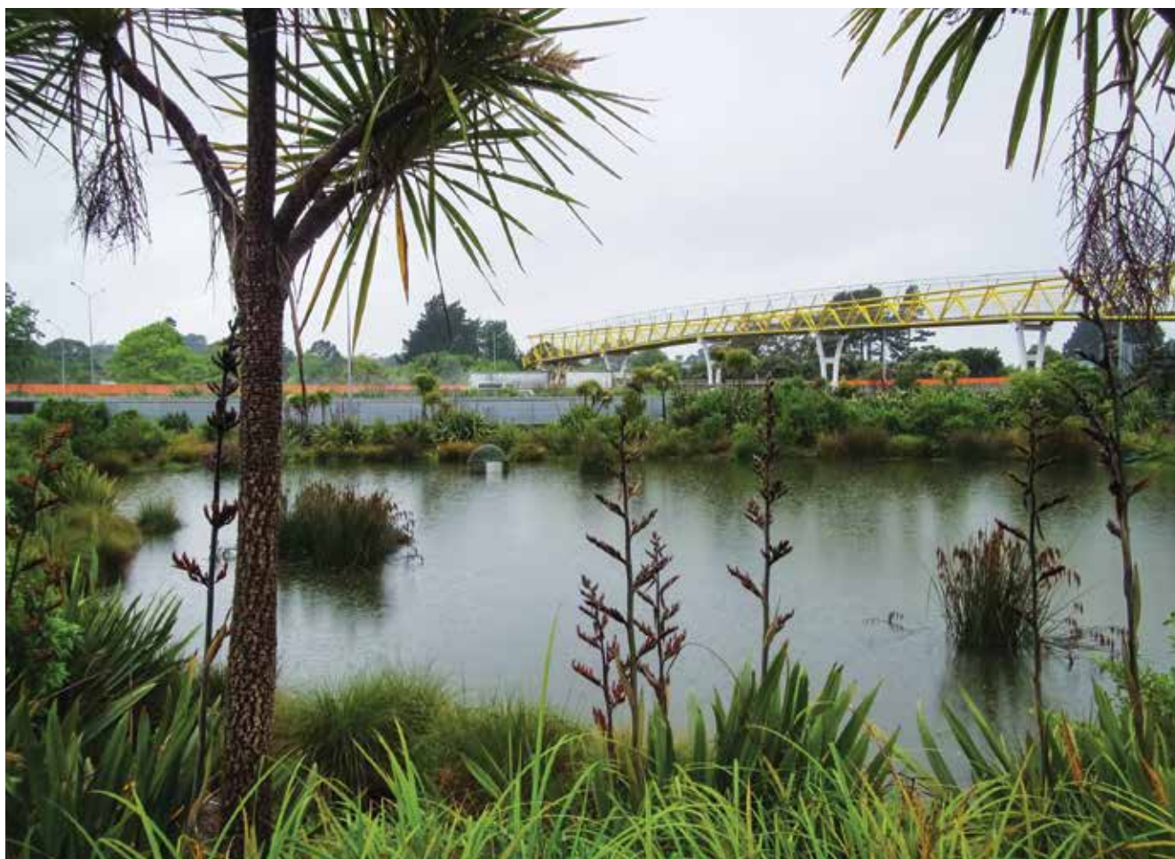
Stormwater treatment devices include engineered ponds and wetlands that allow the contaminants to settle out. (Peter Mitchell, NZTA)
