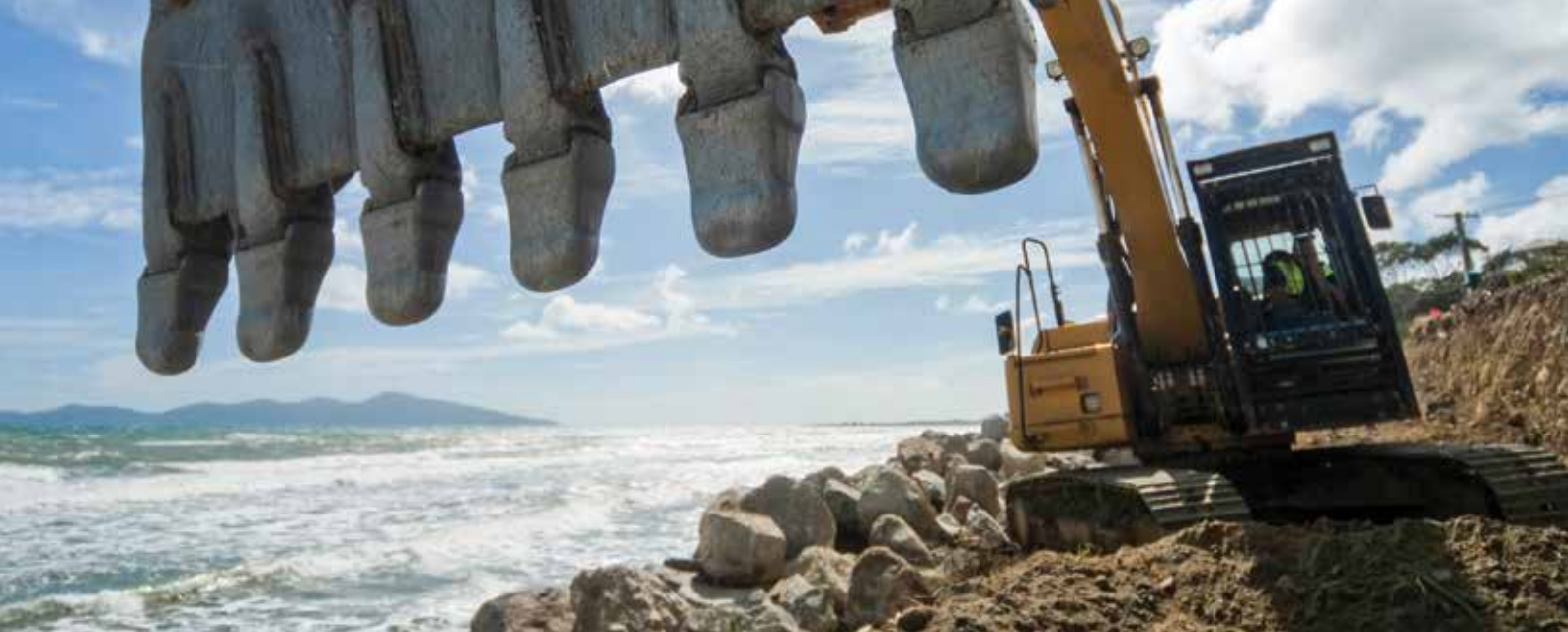
Seawall construction on the Kapiti Coast. (Dave Allen)
