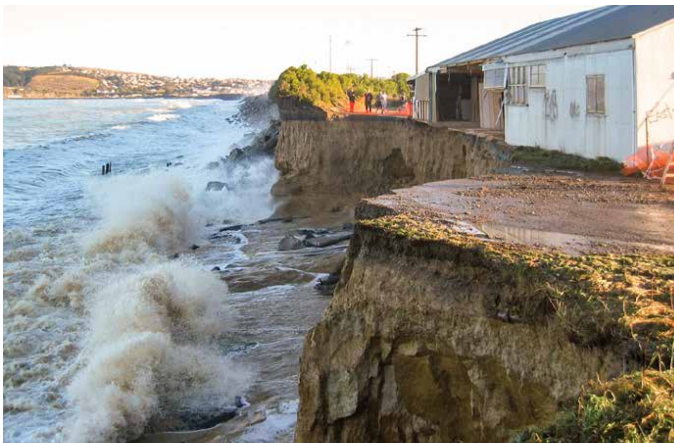
In June 2007, the coastal cliffs at Oamaru lost a lot of ground, including a conservation area for blue penguins and the factory seen here. (Murray Hicks)
