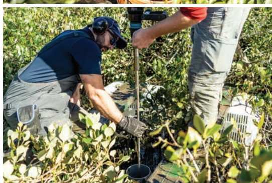
Drilling up to 3m into the mangrove mud, researchers concrete in the poles which will hold the sensitive RSET sea-level rise measuring device. (Lana Young)
