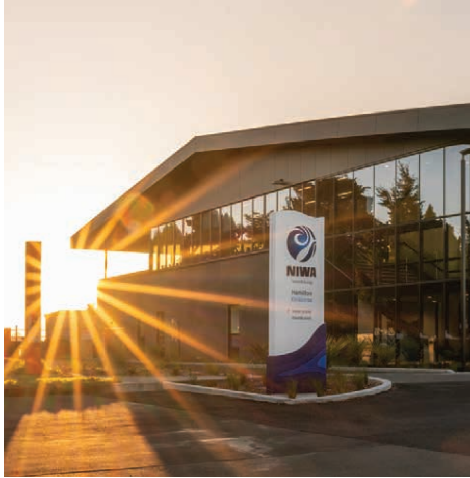
Housing more than 150 scientists, technicians and support staff, NIWA's new 45,000m 2 Hamilton site provides state-of-the-art laboratory and research facilities. [Stuart Mackay]
