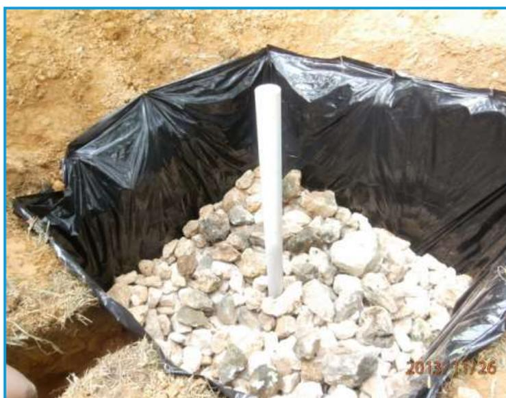
Figure 2. Soak pit under construction.
