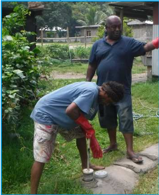
Photo 3. Probing septic tank first chamber for scum and sludge depth.
